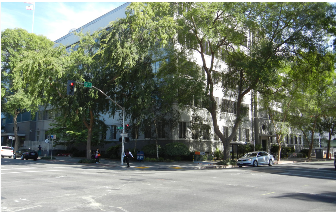
Source: Photograph taken by Ascent Environmental in 2019
